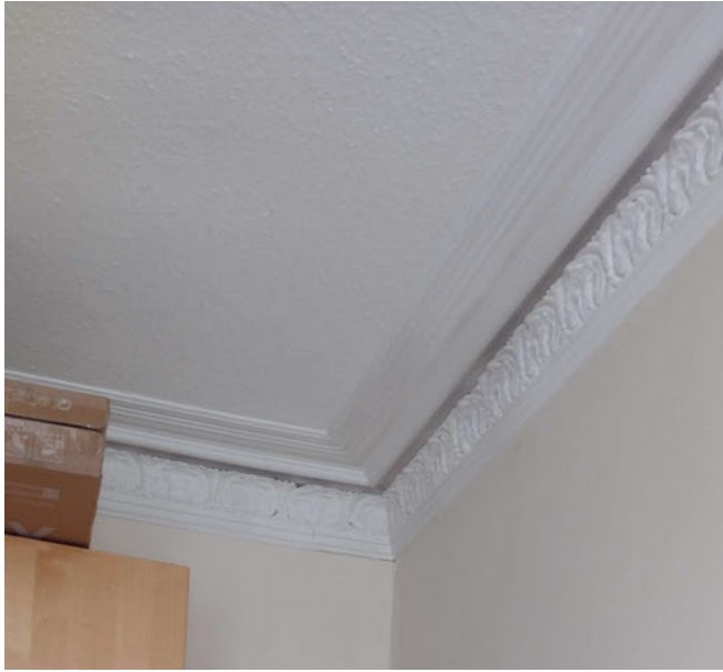
Cornice in bedroom repainted
