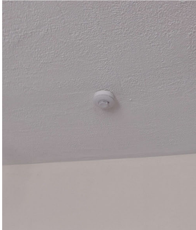
Kitchen living room ceiling
