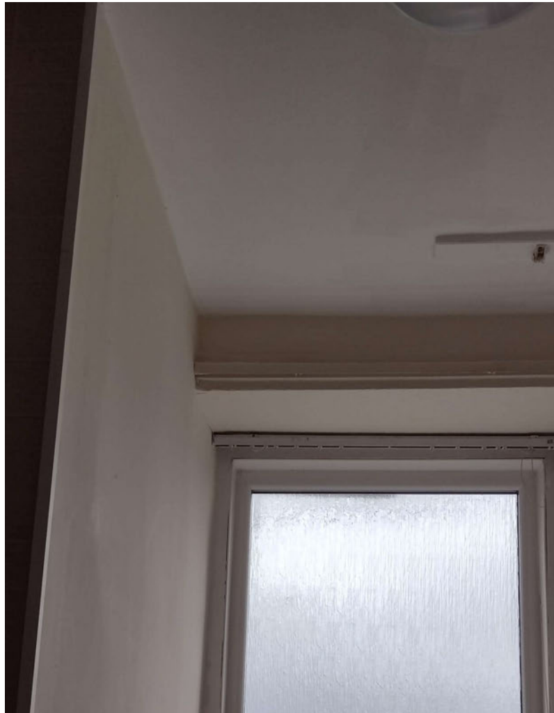
Bathroom wall and ceiling replastered and redecorated
