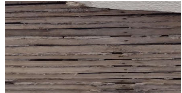
Kitchen ceiling at 19/07/23
