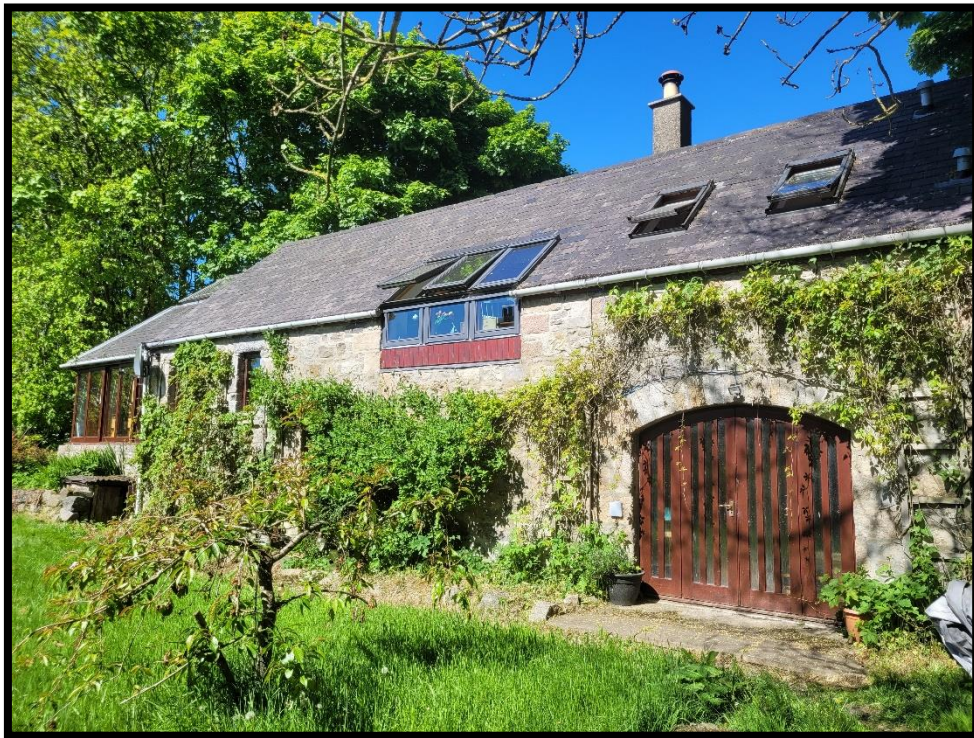
Photograph 1 Front (south east) Elevation.
