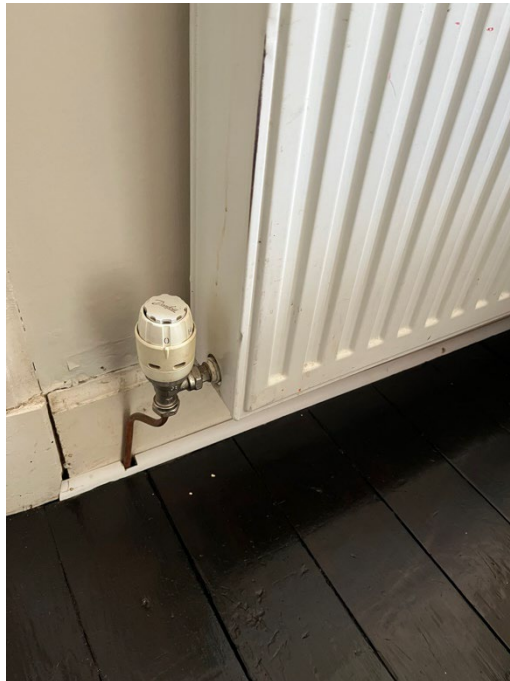
Photograph 14: Living room: flooring and radiator pipework
