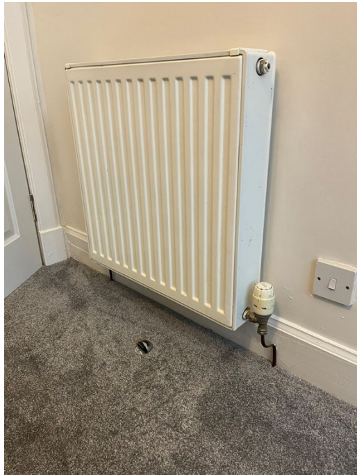
Photograph 16: Bedroom 2: flooring and radiator pipework
