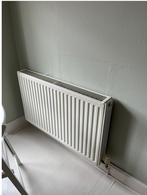
Photograph 17: Kitchen (dining area): flooring and radiator pipework
