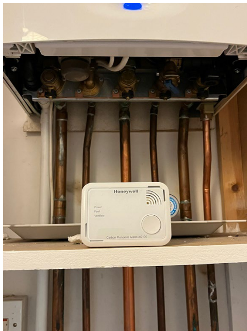
Photograph 11: Bedroom 2: carbon monoxide detector
