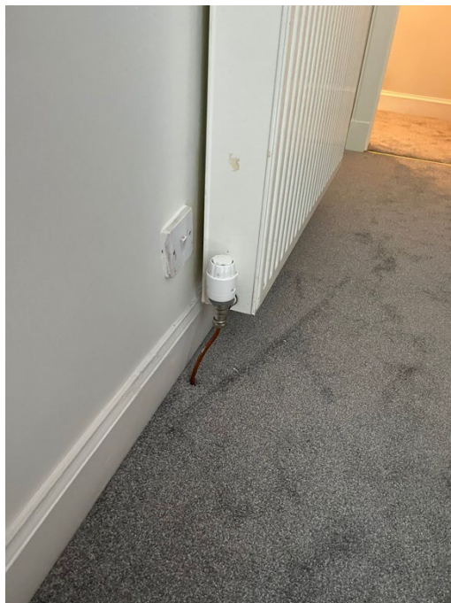
Photograph 15: Bedroom 1: flooring and radiator pipework
