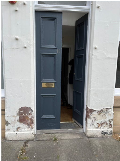
Photograph 2: Front elevation: walls on both sides of front door
