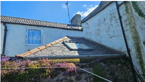
35 Roof over Kitchen.
