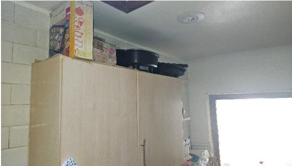
3 View within Kitchen towards separating wall to "coal bunker" area.
