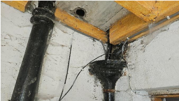
17 Exposed hopper head adjacent to kitchen door within "coal bunker".
