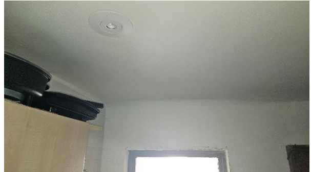
4 Separating wall within Kitchen to "coal bunker" area.
