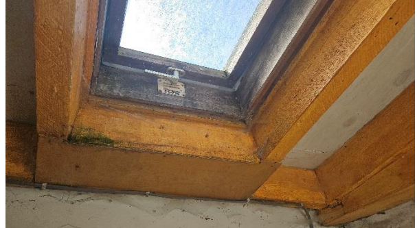
14 "Coal bunker" skylight.
