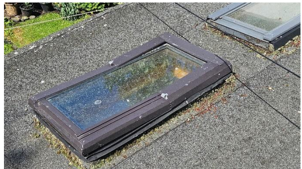
28 Rooflight over "coal bunker".
