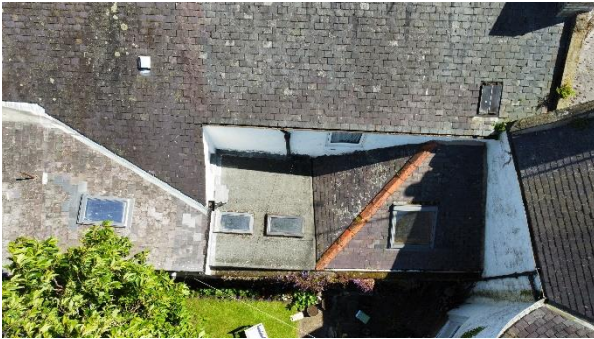
1 Aerial image taken over rear roofing areas.
