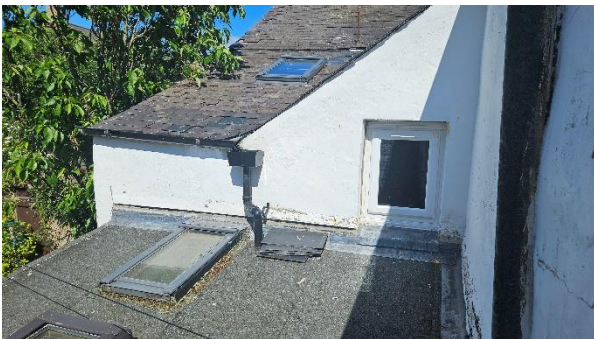
27 View towards gable of adjoining property.
