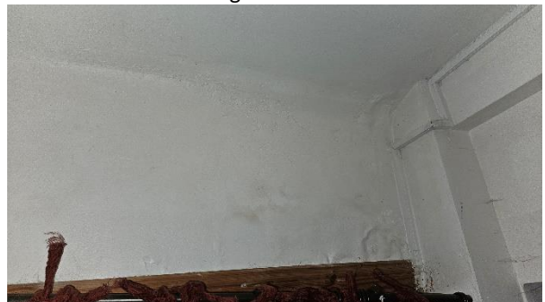
8 Wall area above "coal bunker" door.
