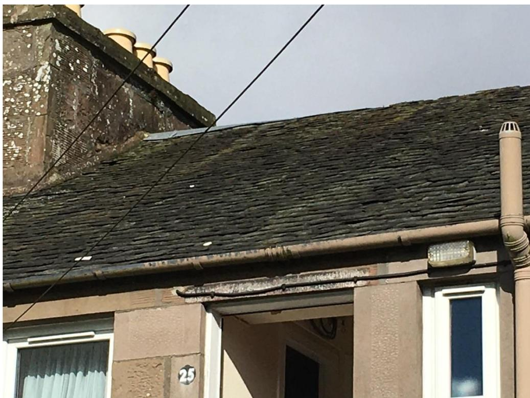
Rear elevation of roof showing slipped/uneven slates and damaged ridge flashing
