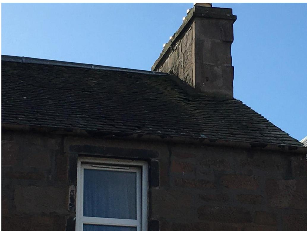
Front elevation of roof showing slipped/uneven slates
