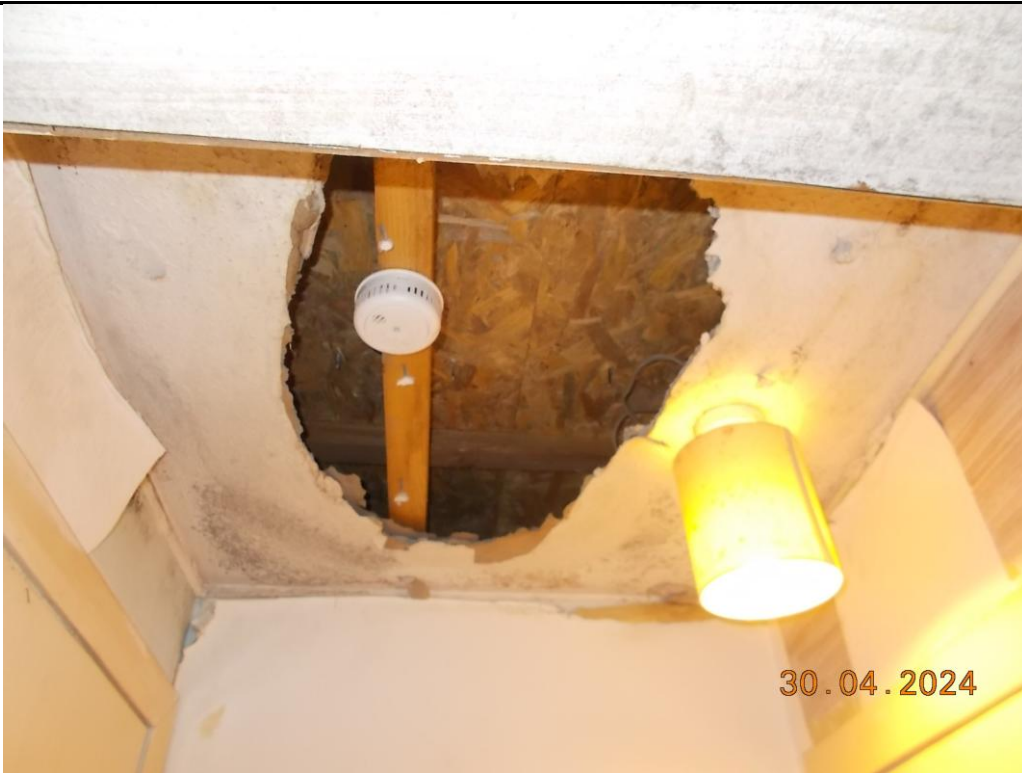
1. Ceiling to entrance vestibule
