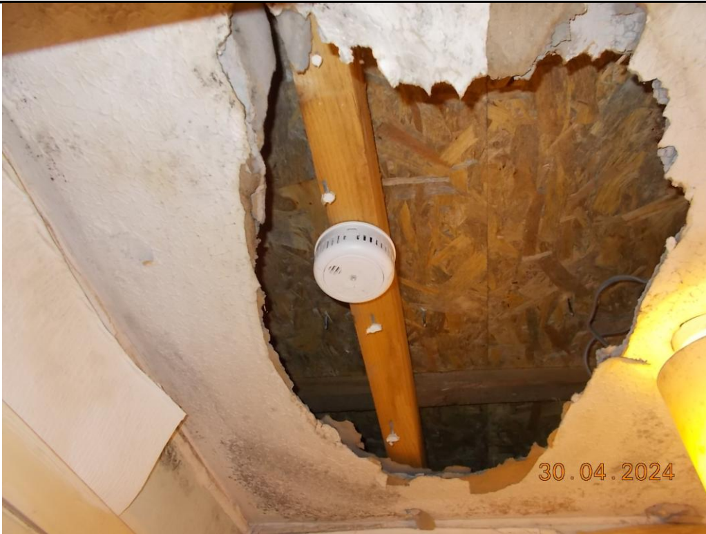
3. Smoke Alarm in Entrance Vestibule
