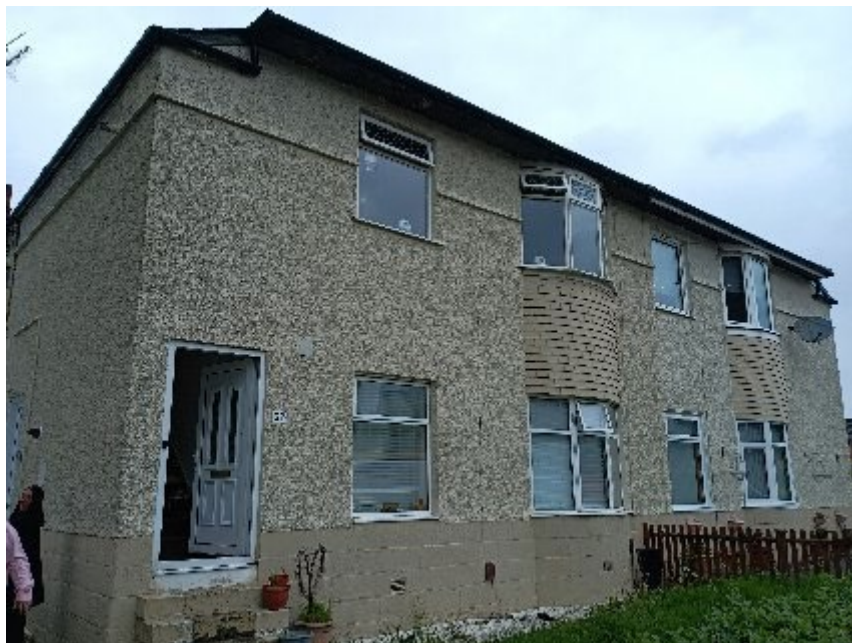
1 Front elevation 32 Kirriemuir Avenue Glasgow
