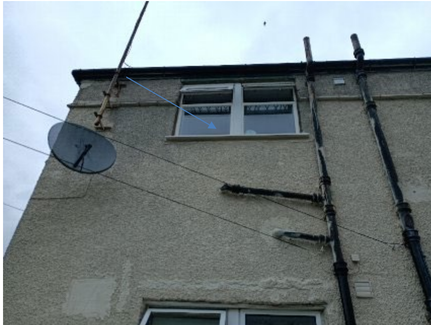
2 South gable kitchen window
