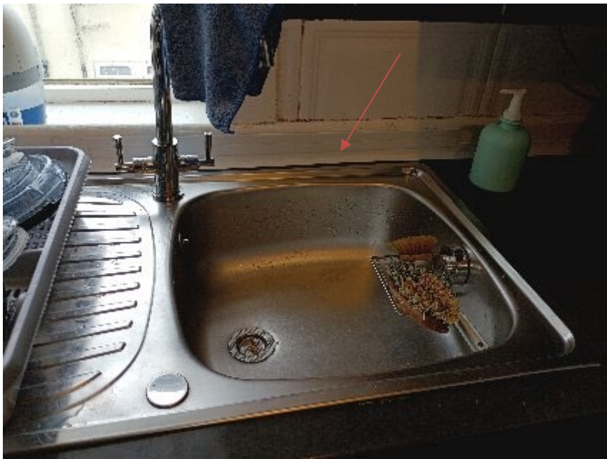
9 The repaired worktop seal behind kitchen sink
