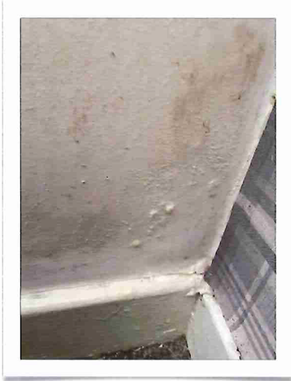
Second Bedroom - High Damp meter readings and staining on walls
