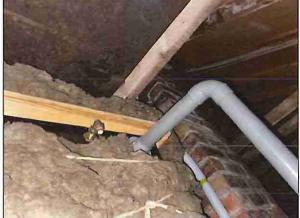
Access to the loft space was limited due to loft insulation covering the loft joists. Unable to identify any woodworm, landlord has advised woodworm has been recently treated by a contractor.
