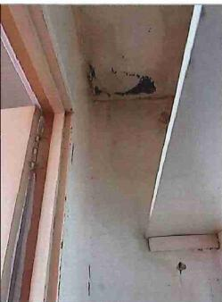
Evidence of historic water ingress visible. No high moisture readings noted on ceiling, walls or in fitted wardrobe.
