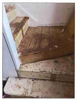
Draught from front door, new seal has been fitted no draught noted at time of inspection. Loose floorboards on stairs have been repaired.
