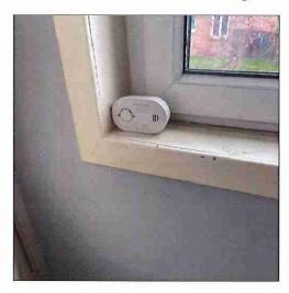
Carbon monoxide monitor has been replaced but not fitted as per guidance.
