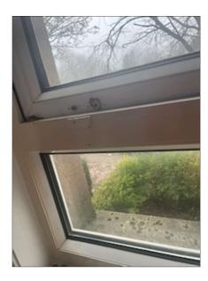
Handle is missing from the rear bedroom window- No repair carried out.
