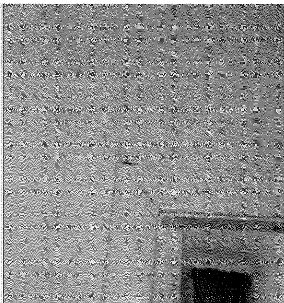
Hall - crack through bathroom door frame and wall above, door frame not square
