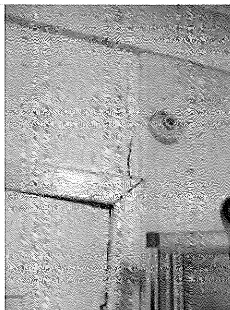
Bathroom - party wall between hall and bathroom - severe settlement crack through door frame and wall above
