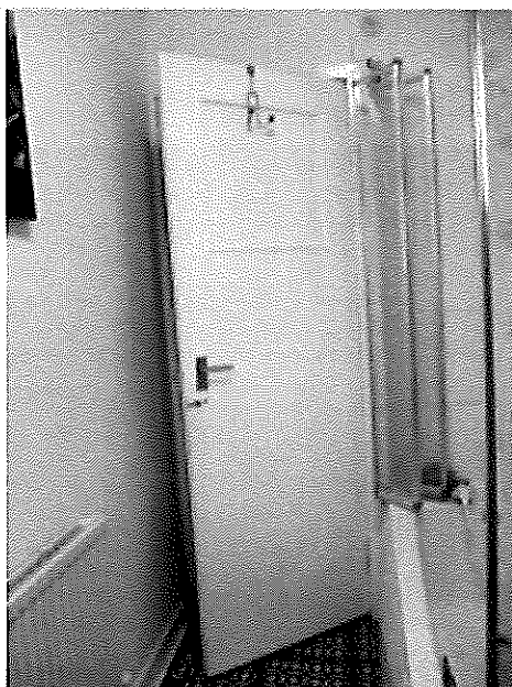
Bathroom door - misaligned and does not close/ floor sloping and door frame not square
