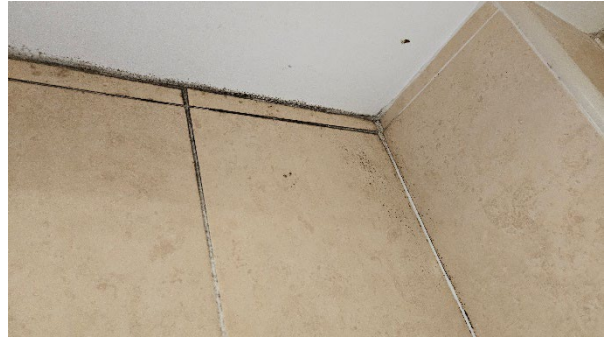
12 Mould within Bathroom over external wall.
