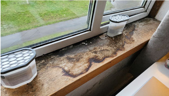
3 Water staining to timber sill (Living Room).
