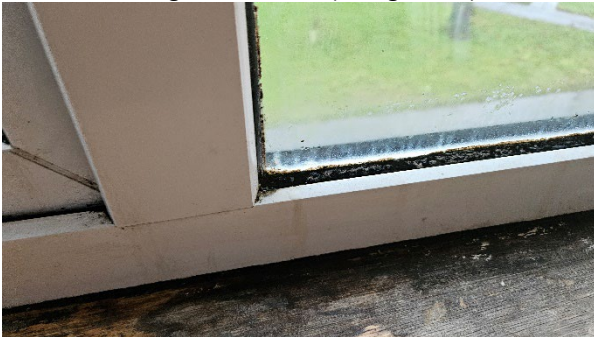
5 Mould growth at gasket seals of window (Living Room).
