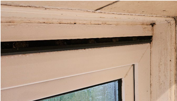
13 Condensation droplets at window frame.
