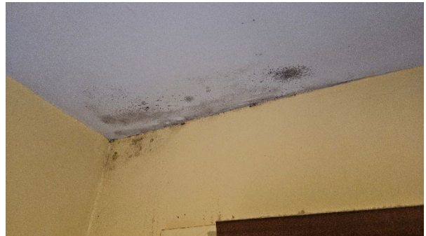
16 Mould growth at external wall to ceiling junction within Kitchen.
