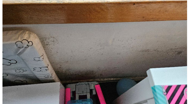
4 Mould growth below Living Room window.
