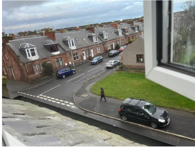
Photograph 8: Guttering – street elevation
