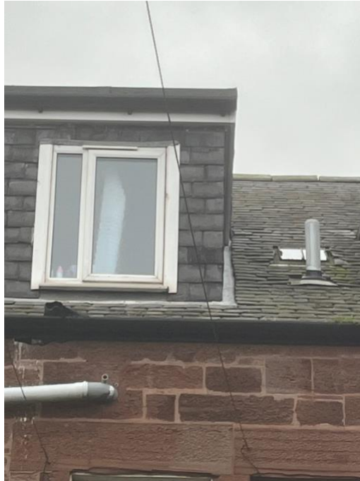
Photograph 9: Entrance elevation: guttering
