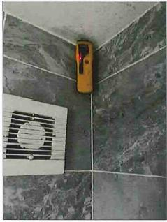
Unable to test mechanical extract fan as no electricity in house. No evidence of mechanical ventilation vented externally. High moisture readings noted.
