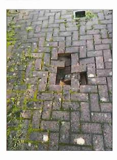
Sections of the mono bock drive has collapsed at the rear of the driveway.
