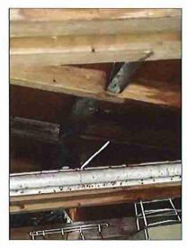
Felt roof has perished in part, daylight visible and water ingress noted.
