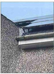
The chimney pot appears to have been removed, evidence of flashing damaged in sections and slipped, broken slates noted.
