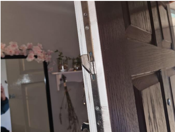
9 2-hook multipoint locking system to main entrance door.
