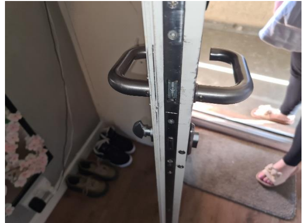
8 2-hook multipoint locking system with defective central latch to main entrance door.
