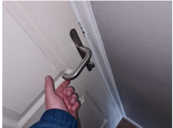
14 Loose lever handle to main entrance door.
