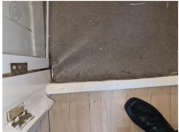
22 Poor perimeter detailing to floor and wall junctions of wet room area.
