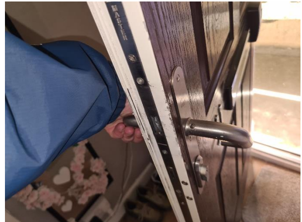
10 Defective central latch to main entrance door.
