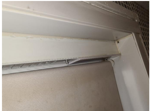
18 Kitchen trickle vent boxing with retrofit capping cover plate.
