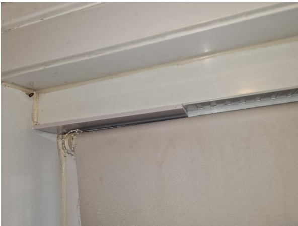
17 Kitchen trickle vent boxing with retrofit capping cover plate.
