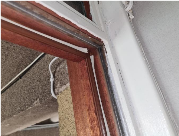
13 Primary and secondary seals to entrance door.
