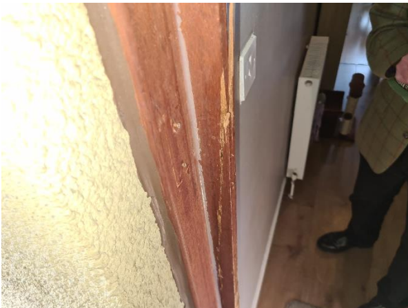
11 Timber external door stop to main entrance door split.
