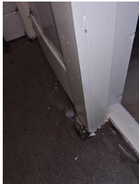
24 Poor perimeter detailing to floor and wall junctions of wet room area.
