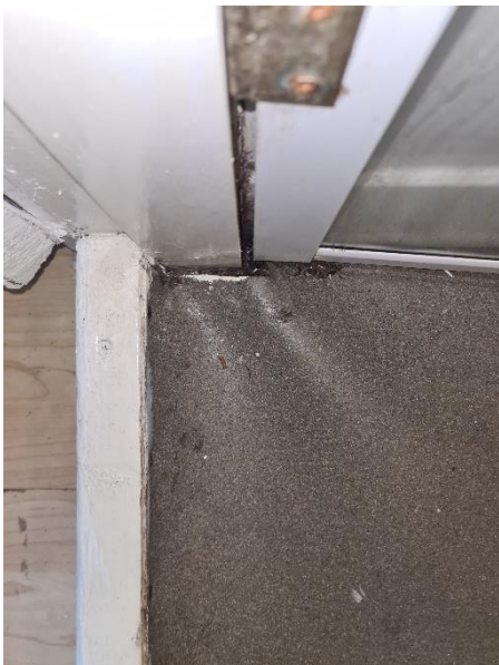
23 Poor perimeter detailing to floor and wall junctions of wet room area.
