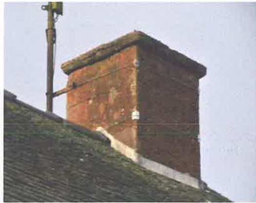
Chimney head 4 December 2019
