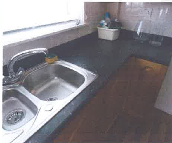
Replacement worktop 17 March 2020
