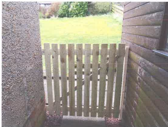
Replacement timber gate 17 March 2020
