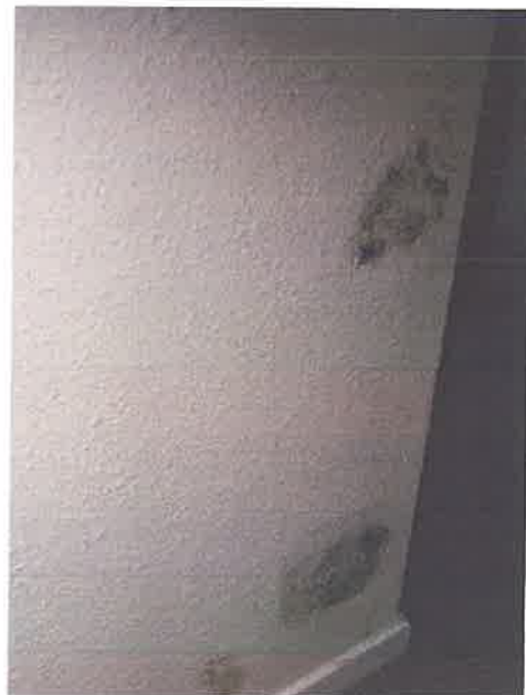
Mould and damp in hall wall 4 December 2019
