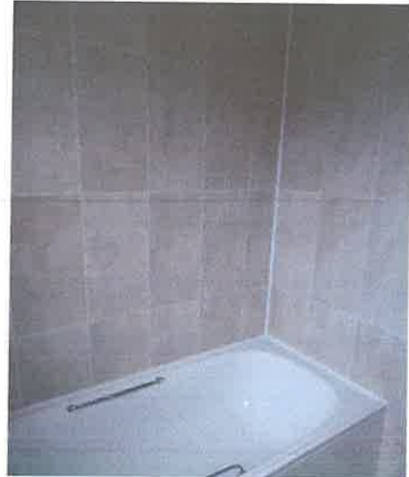
Replacement lining 17 March 2020
