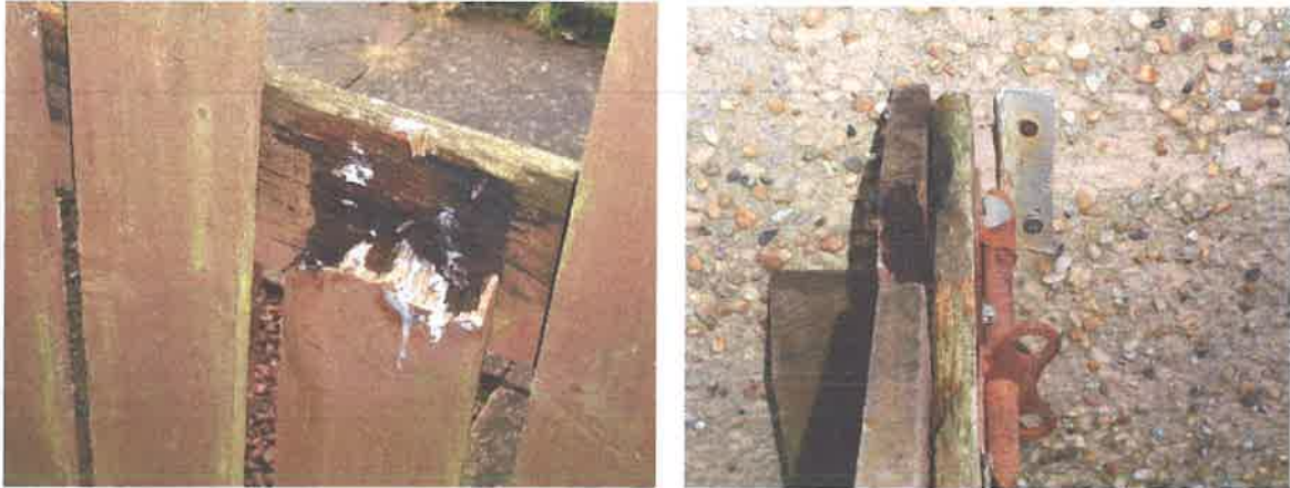
Projecting nails, broken spar and defective closing mechanism at garden gate 4 December 2019
