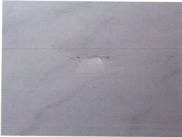
Damaged wet wall lining 4 December 2019
