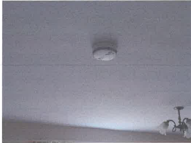
Ceiling mounted smoke detector in living room 17 March 2020
