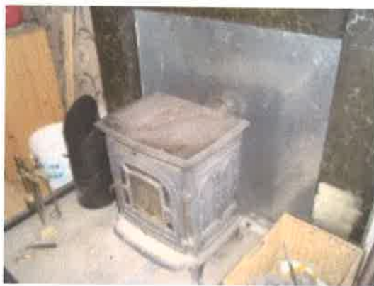
STOVE – FLUE LINER
