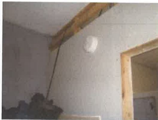
HEAT DETECTOR – KITCHEN
