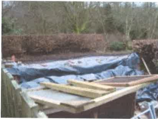
FRONT BOUNDARY UNDER REPAIR
