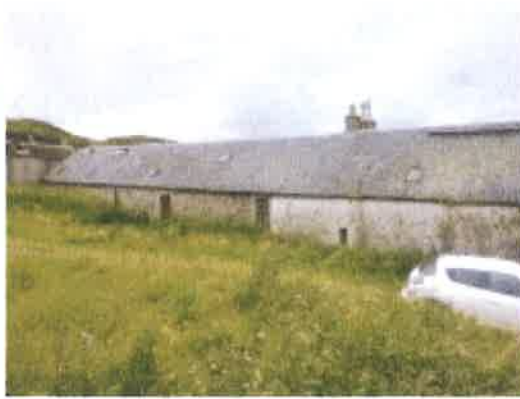
OUTBUILDING – REAR ELEVATION
