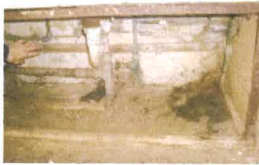
STOPCOCK UNDER SINKS
