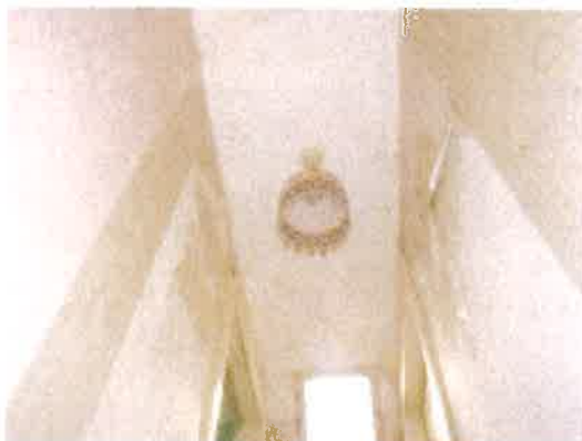
UPPER LANDING CEILING
