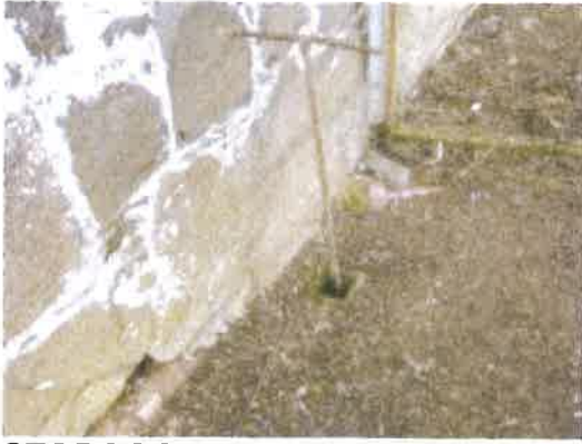
STOPCOCK AT OUTBUILDING
