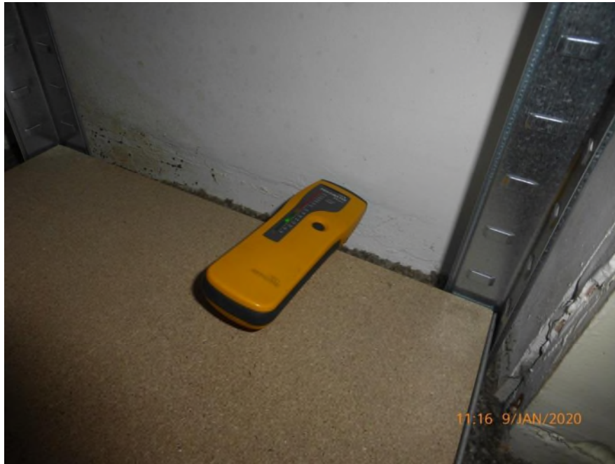
Damp meter reading
