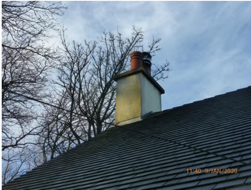
Replaced roof covering and chimney pot.
