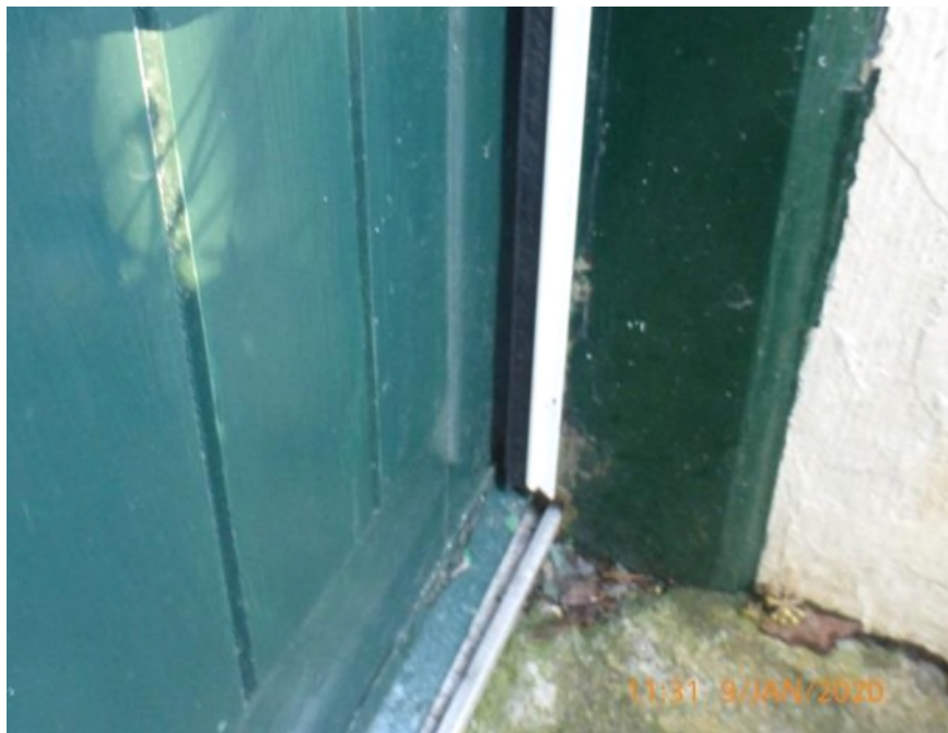
Gap between draughtproofing strip and the back door
