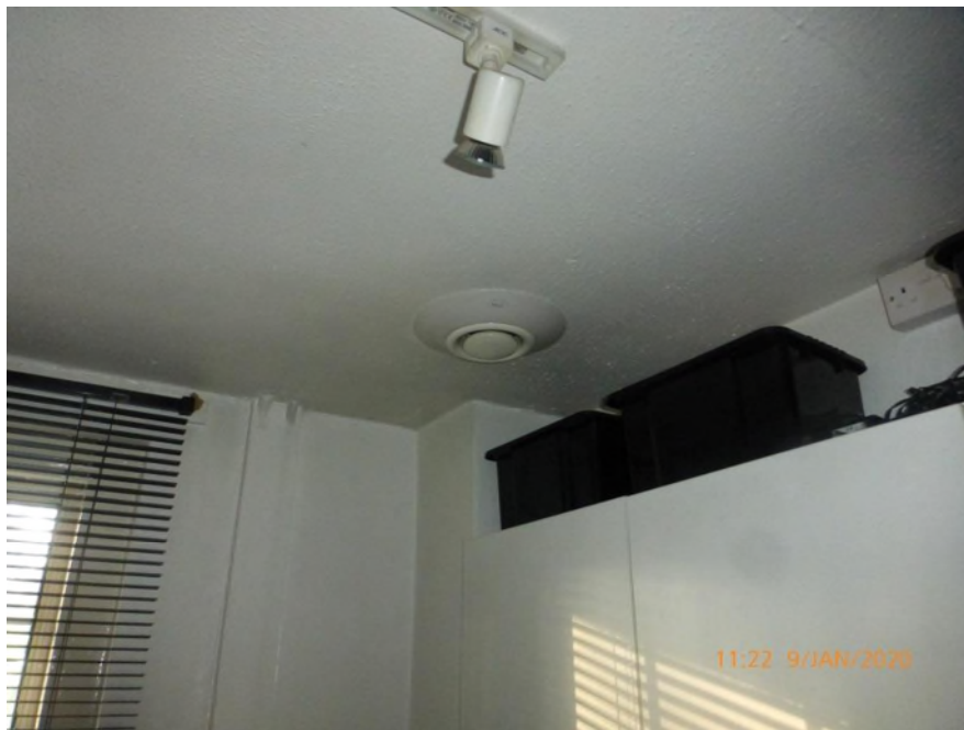
New vent in the kitchen
