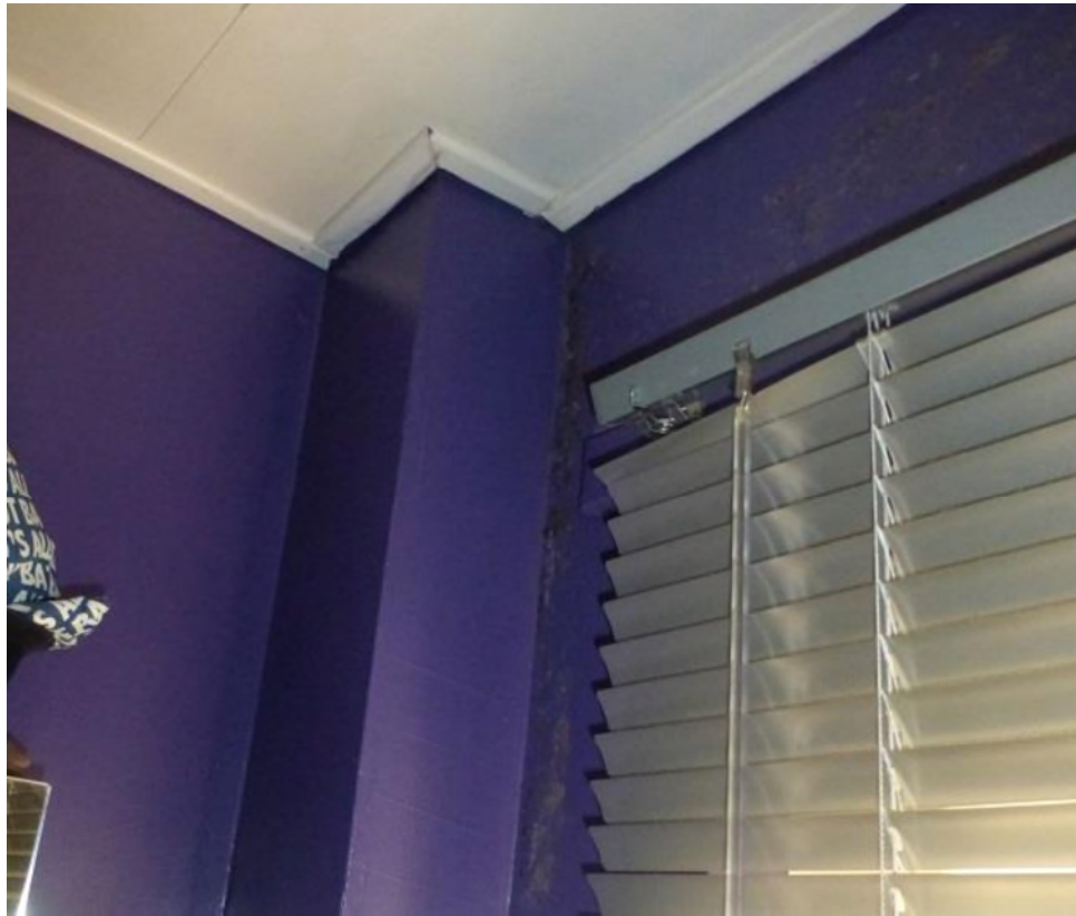
Mould in the shower-room
