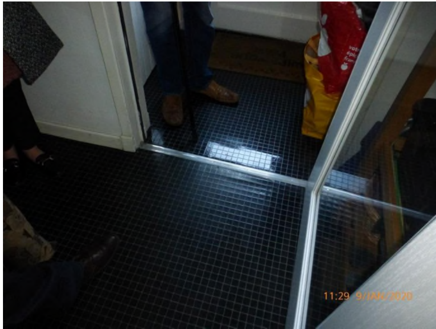
Replaced floor covering inside back door.
