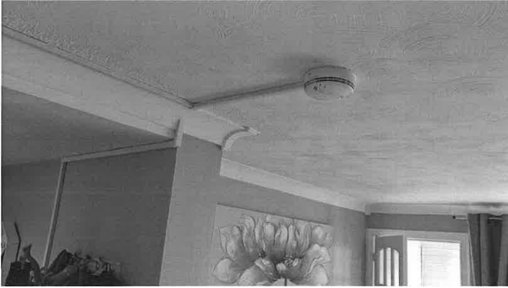
5 The new hard-wired smoke detector in the living room
