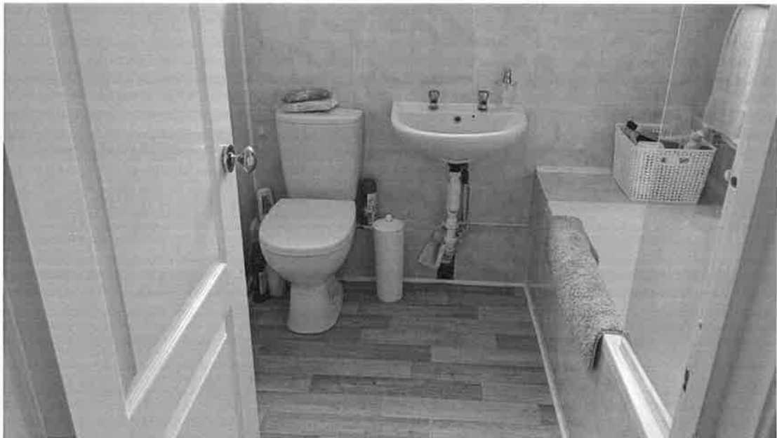
4 The new bathroom fittings
