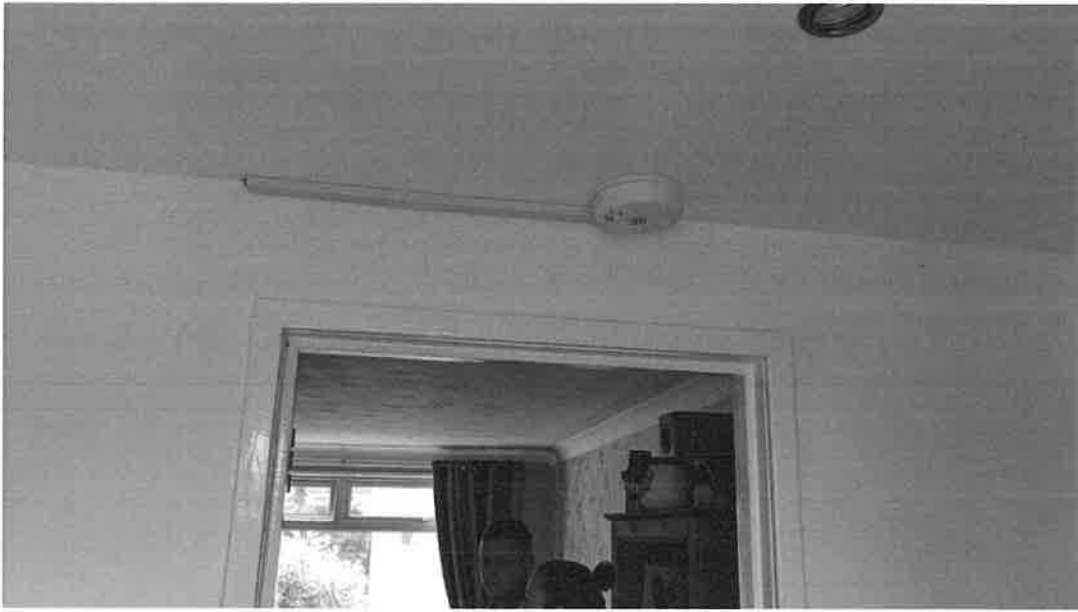
3 The new hard-wired heat detector in the kitchen
