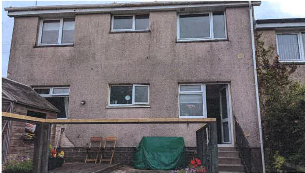
1 Rear elevation of 80 Hazel Road
