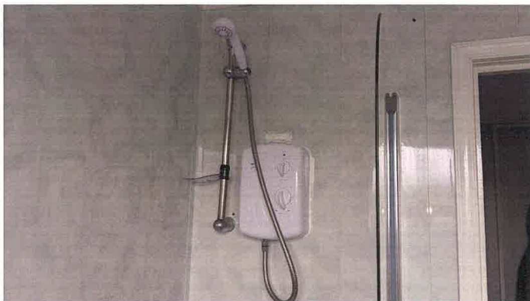
2 The new shower unit in bathroom A Cowan
