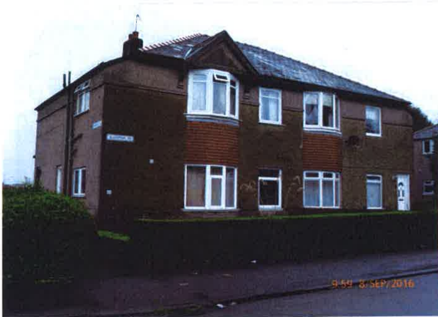
First Floor Front
