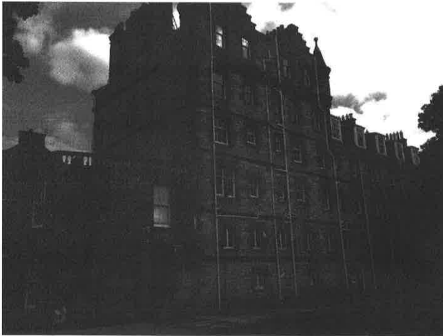
Rear of the building
