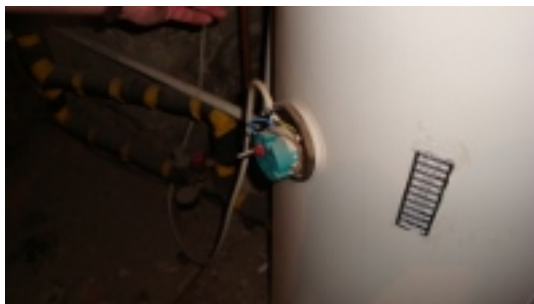
BOILER-MISSING CAP AT IMMERSER
