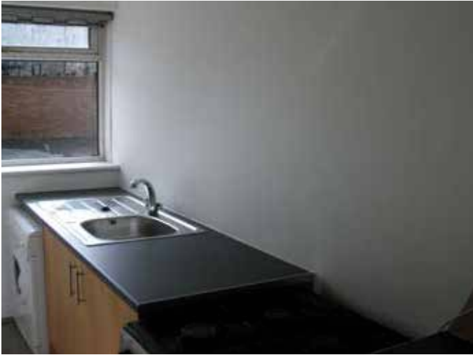
Kitchen looking to rear
