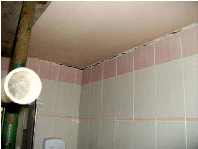
Bathroom looking to hall showing propping and cracking
