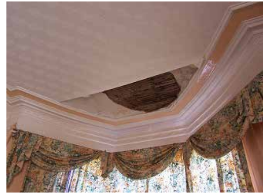
Damage caused by roofing issue at a property
