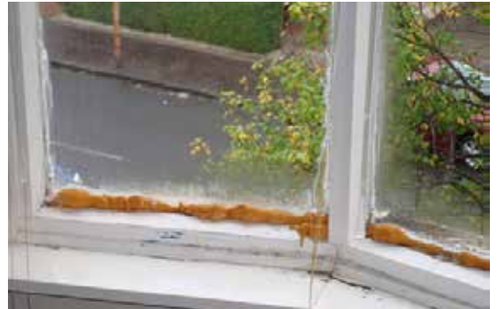
Window defects at a property at time of inspection
