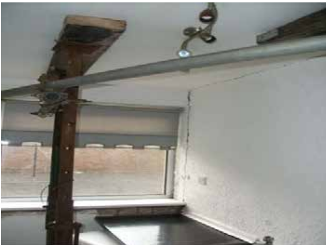
Kitchen looking to rear showing propping and cracks at the wall and ceiling
