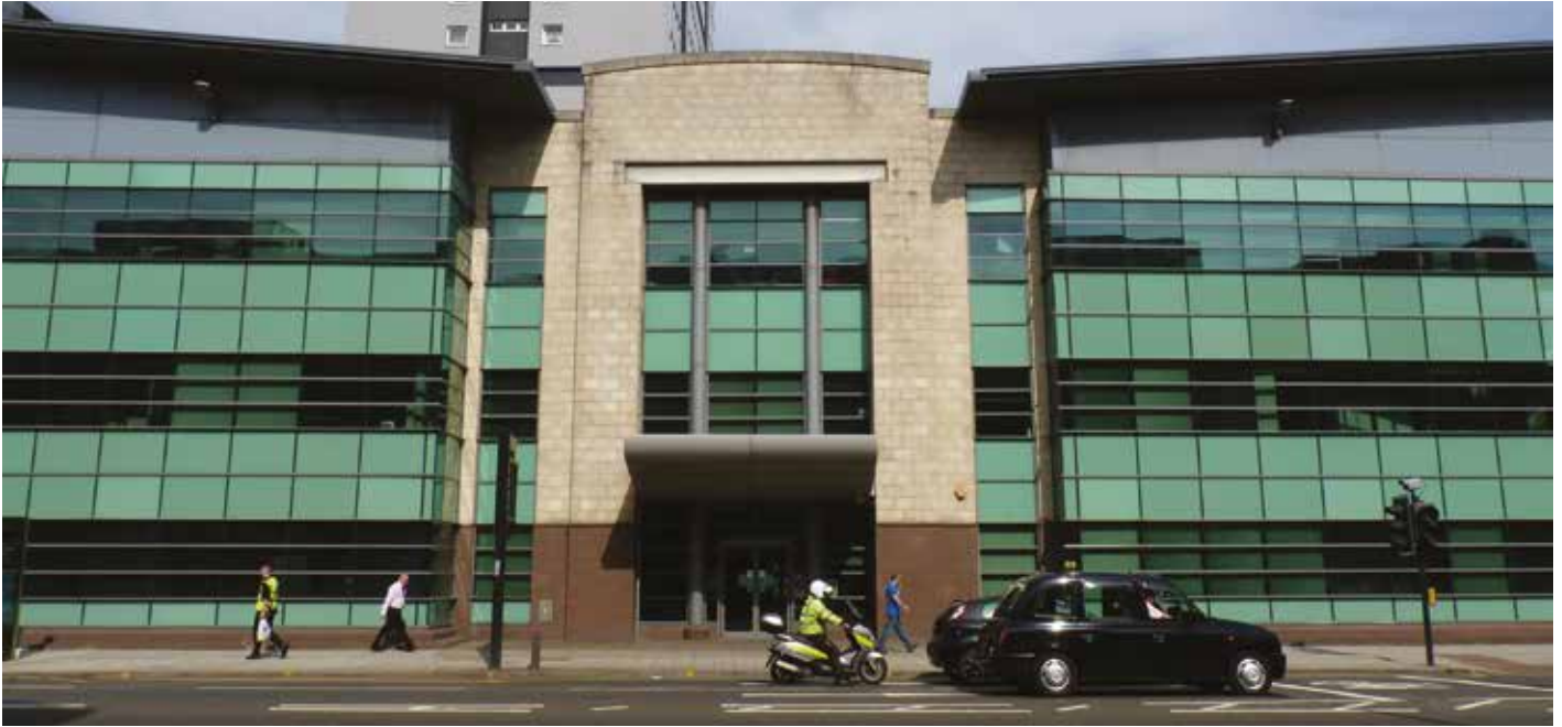
Prhp and hohp offices at Europa Building, Argyle Street, Glasgow
