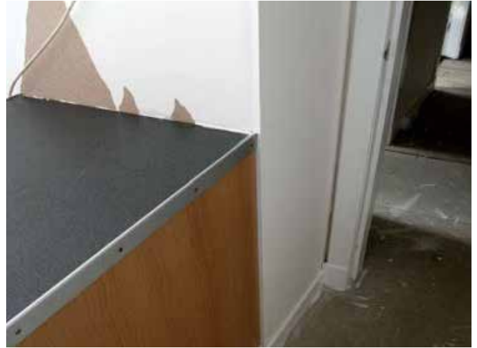
Kitchen showing lower wall at corner
