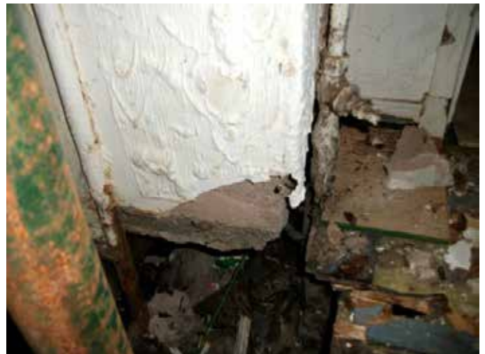
Kitchen showing lower wall at the corner
