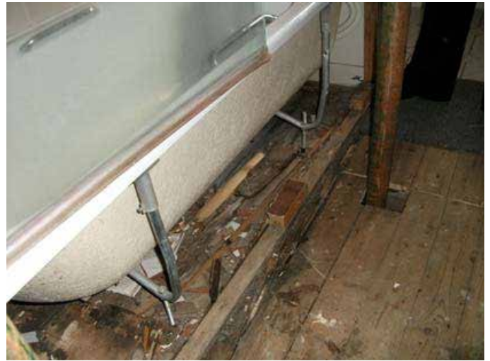
Bathroom showing floor at bath
