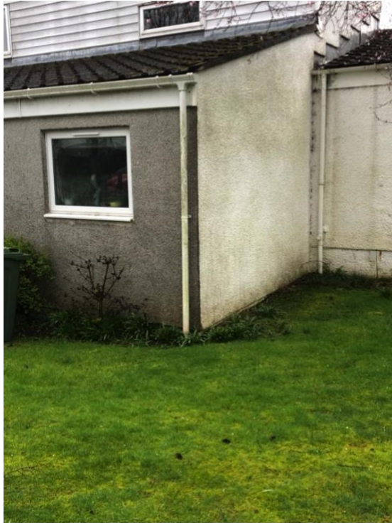
Photo 20 – Re-rendered section of wall
