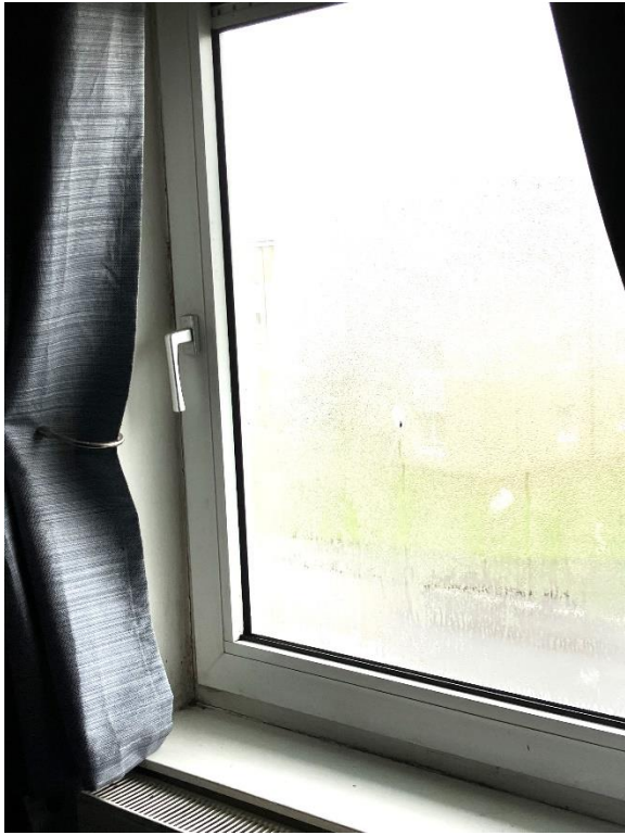
Photographs 7 & 8 :- Condensation and mould around bedroom 2 window
