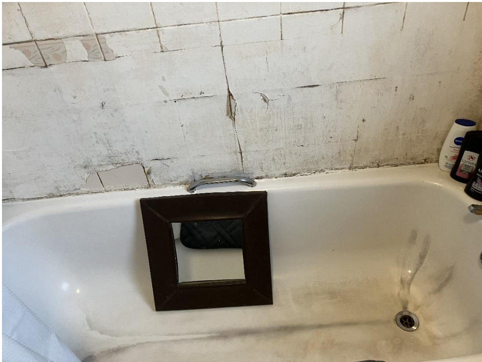
Photograph 21:- Significant mould and flaking paint around bath
