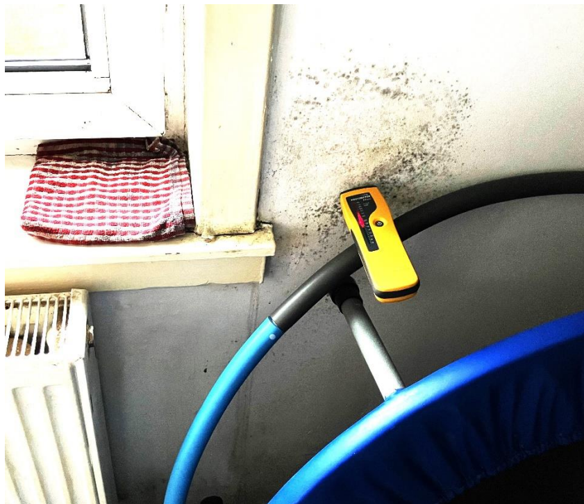
Photographs 9 - 12:- Significant damp around bedroom 3 window
