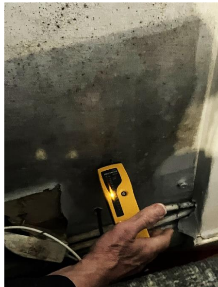
Photographs 23 & 24:- Significant damp staining, mould and defective plaster around random wiring at front wall of living room.
