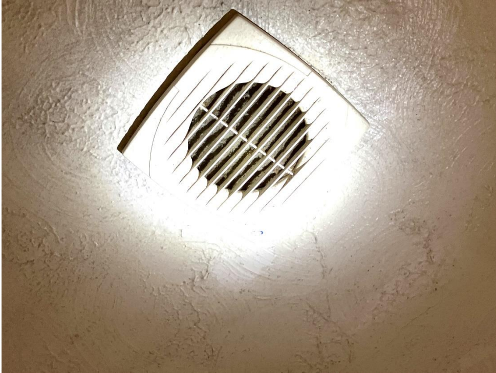
Photograph 20 :- Choked and ineffective electric ventilator in bathroom ceiling
