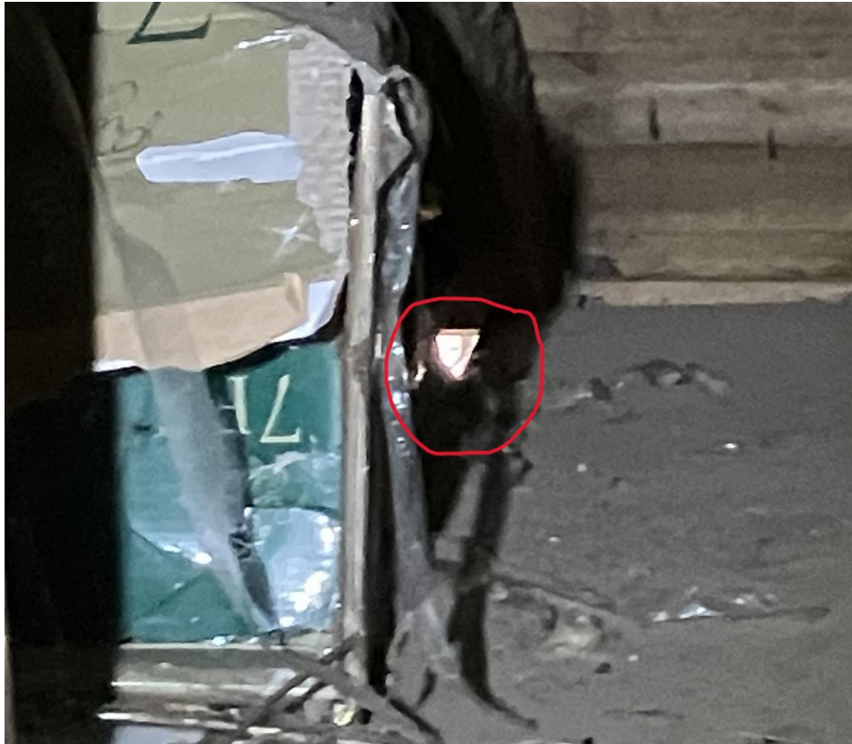
Photograph 27:- Circled area is a hole in roof/eaves, visible daylight, and is likely access for nesting birds.
