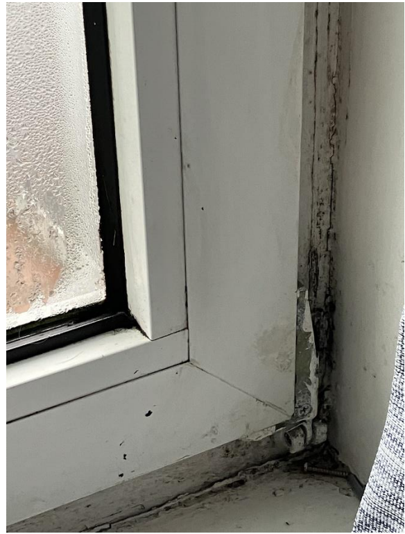
Photographs 7 & 8 :- Condensation and mould around bedroom 2 window
