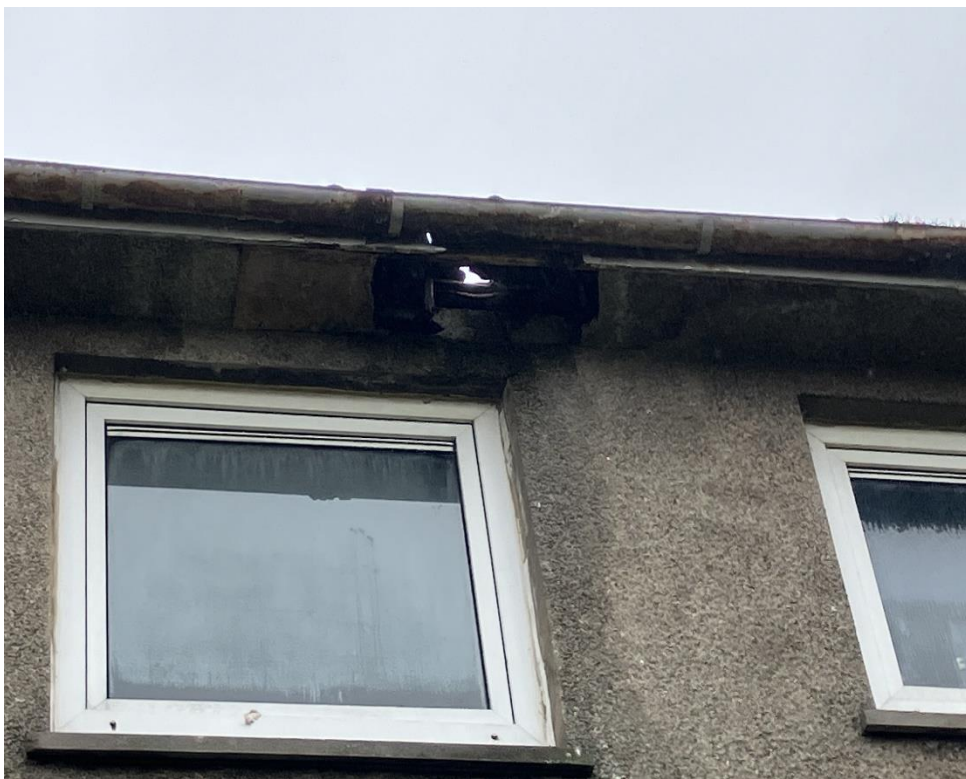
Photograph 27:- Circled area is a hole in roof/eaves, visible daylight, and is likely access for nesting birds.
